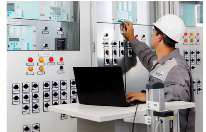
7 Works on site
