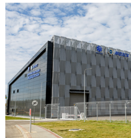
EKRA introduces the first fully digital substation Medvedevskaya in Russia
